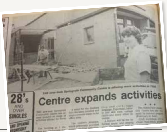
Bev Douglas in front of the Centre during extension works. Dandenong Journal, 5 February 1990.
